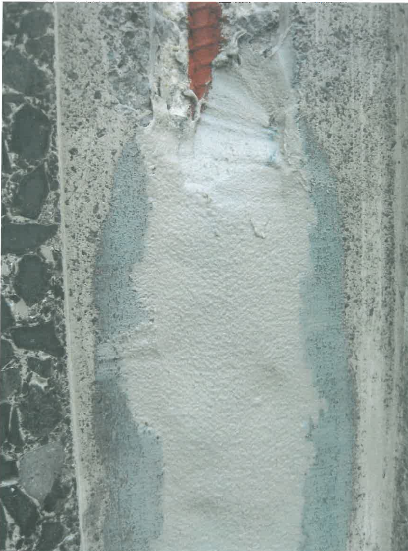
Fig.5 - Sample of treated steel and concrete mortar repair.
