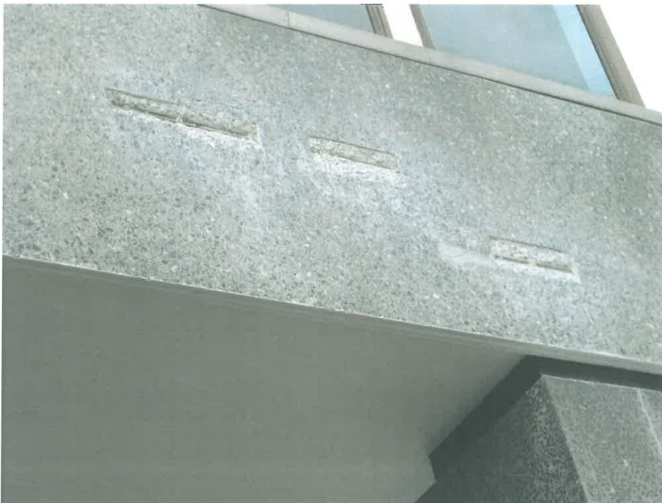
Fig.3 - Horizontal reinforcing alignment.
