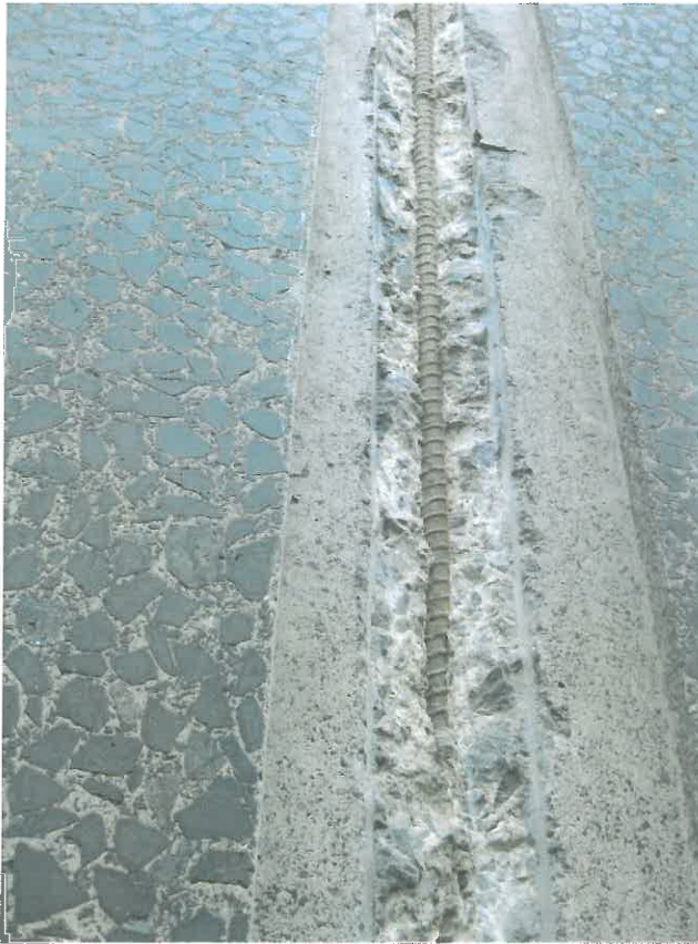
Fig.2 - Vertical reinforcing alignment.
